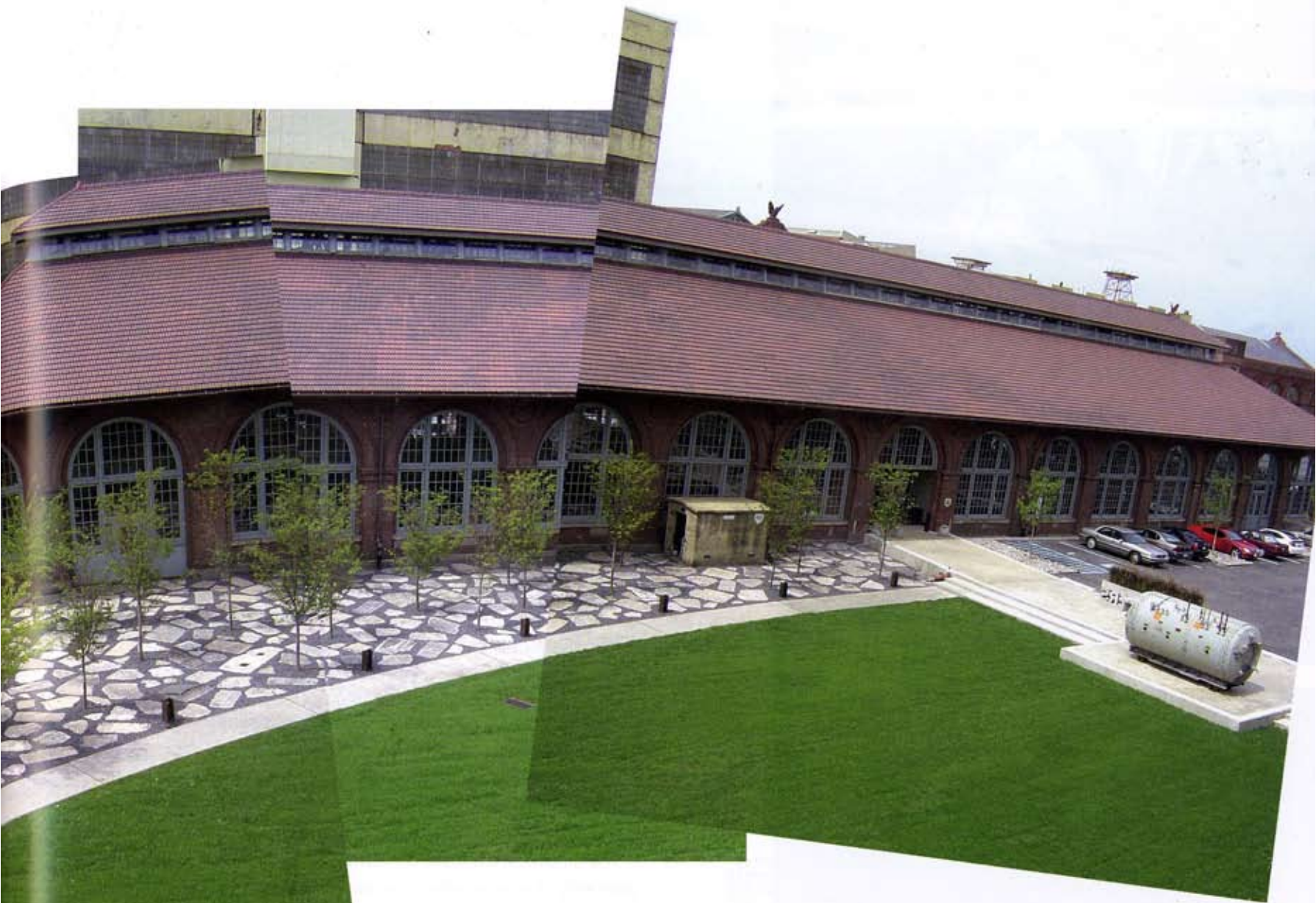
For more than a century, Navy men and women labored on thick slabs of concrete crafting huge ships. That historic surface was salvaged and reconfigured as a terrace at Urban Outfitter's headquarters.
